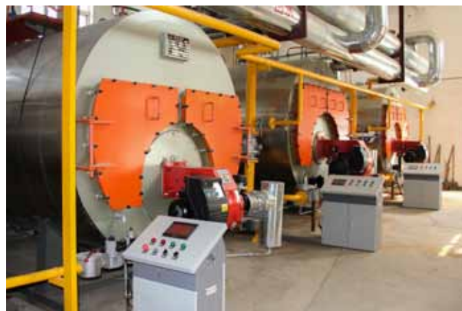
2x BLU 4000 FGR on 2x 2,8 MW hot water boilers 1x BLU 2000 FGR on a 1,4 MW hot water boiler
